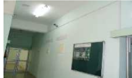
CCTV CAMERA INSTALLED IN THE LIBRARY THIS YEAR
